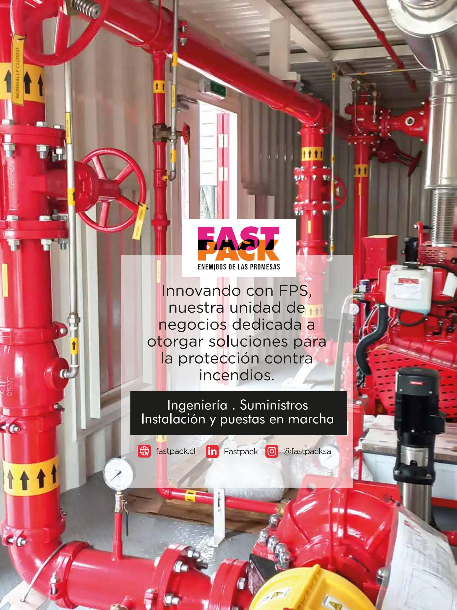
The background image shows a fire pump room with extensive red piping, valves, and a fire pump engine. A pressure gauge is visible on the left. The room has a window and a door in the background.
